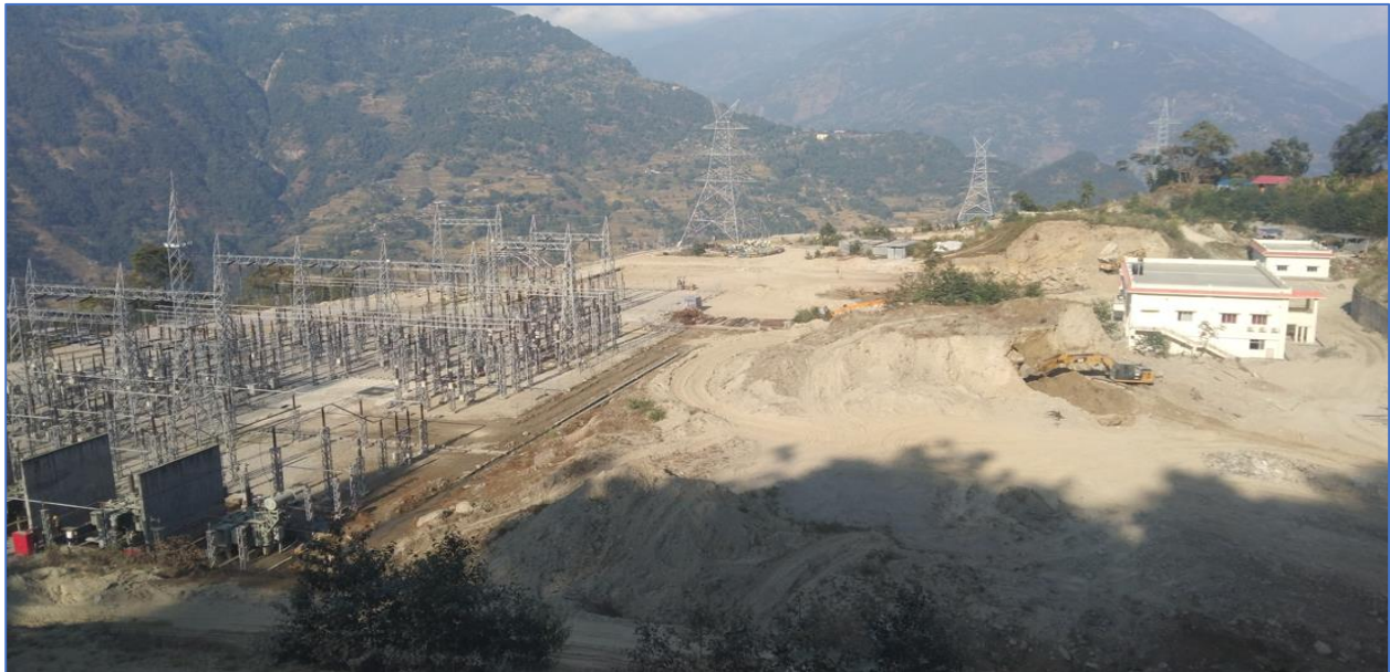
Completed 220/132/33 KV Substation of NEA in Dhungesaghu (Hangpang)
