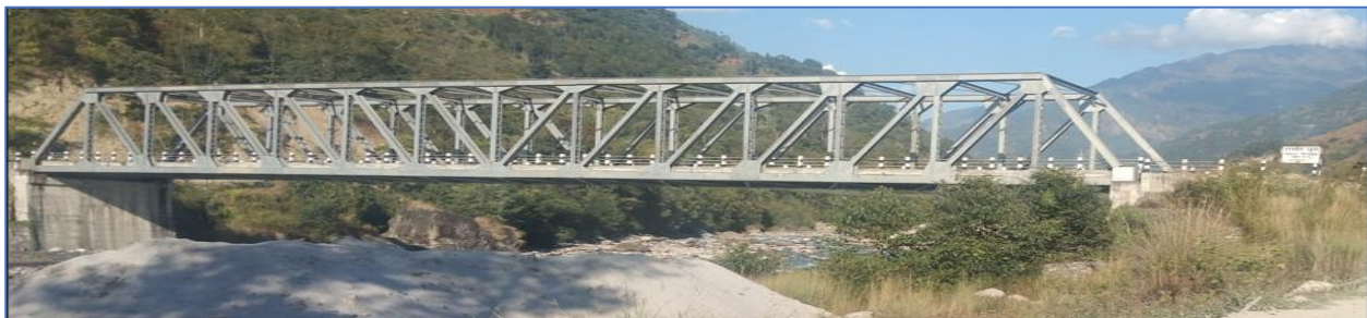
Motorable bridge in headworks
